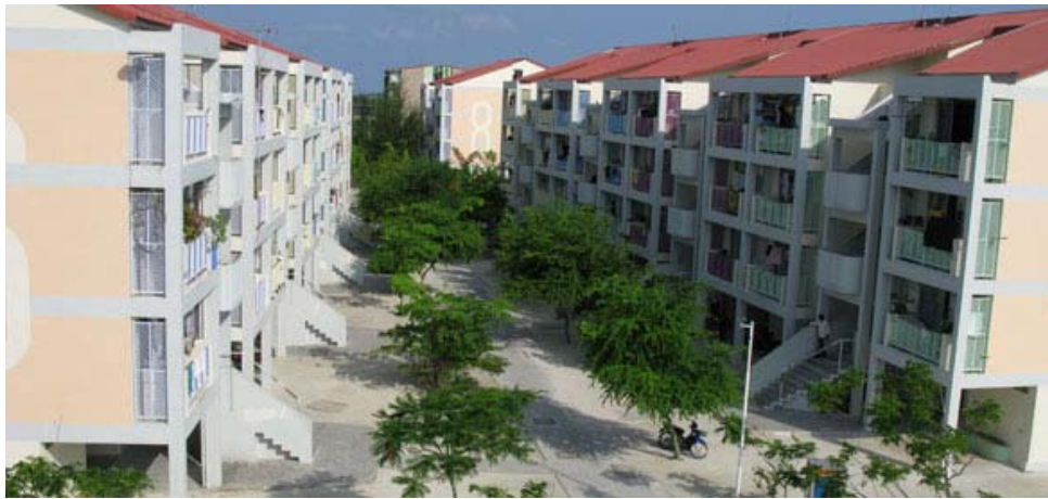
Apartment blocks in Hulhumalé'
